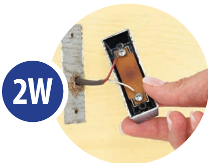
Upgrade Existing 2-Wire Systems
